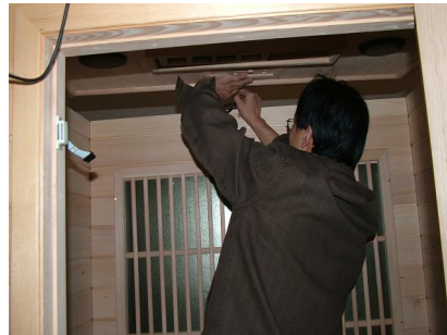
FIG-13 Leading the wires of heaters onto the board through the corresponding hole
